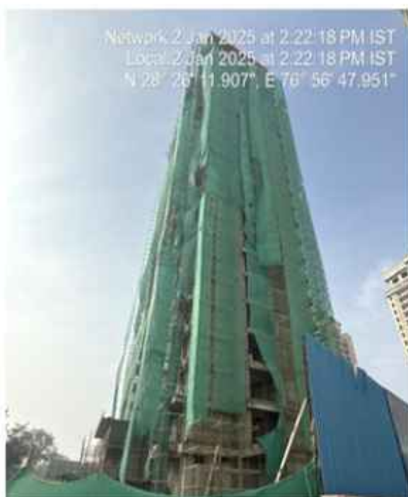
Construction site fully covered with Dust Screen
