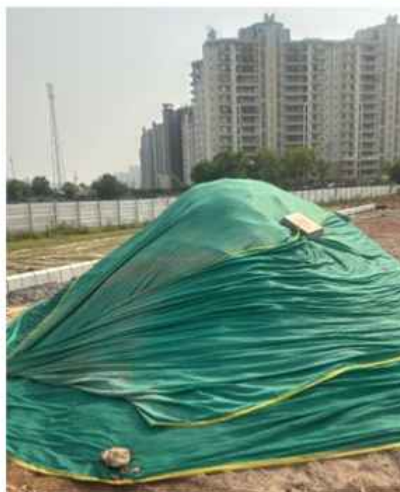
Construction material covered with Dust Screen
