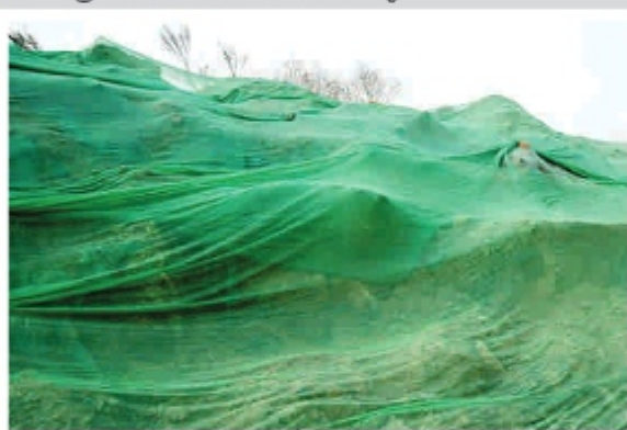
Proper covering of stacked construction materials
